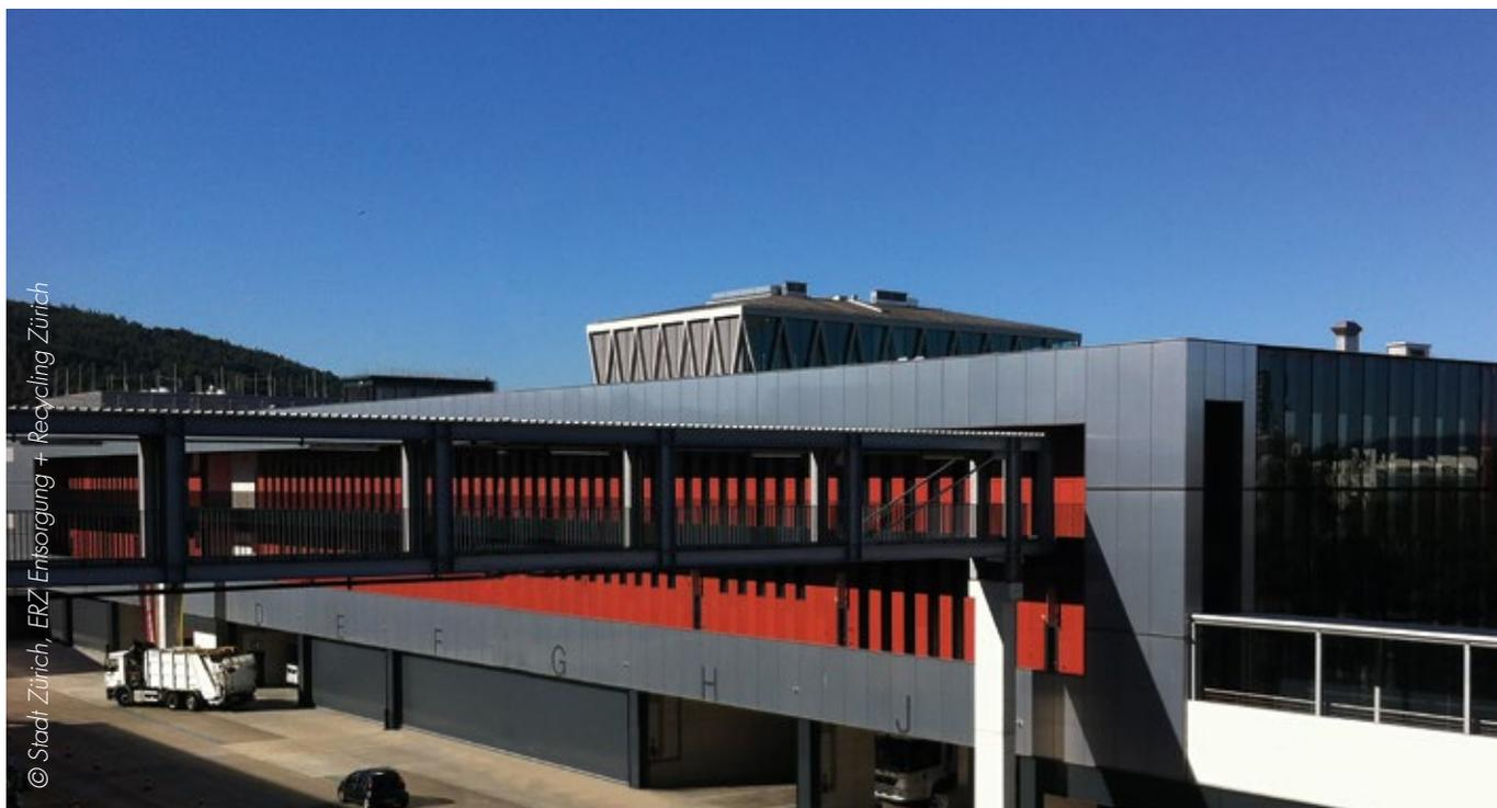
Heat and electricity is produced from refuse around the clock at the Hagenholz waste incineration plant. The administration staff now also work in a new logistics building on the same site. In line with its energy and environmental targets, the city of Zurich is deeply committed to higher energy efficiency and therefore designed the building to meet the stringent Minergie P-Eco standard.
