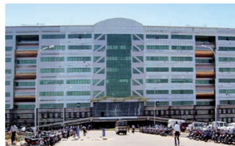
ETL Building, India
